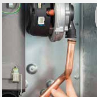
Removal of the gas pipe
