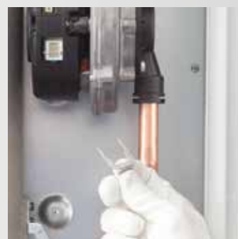
Releasing of the gas pipe from fan
