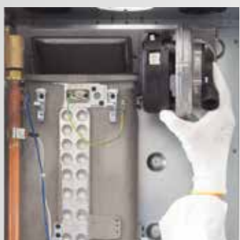
Removal of the complete combustion system
