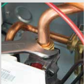
Releasing of pipe from the gas valve
