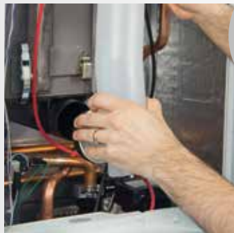
Removal of the smoke manifold
